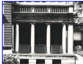
Exterior of existing building
